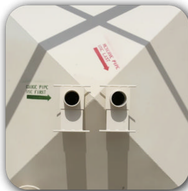
4" Drain Pipe and 4" Reserve Pipe
